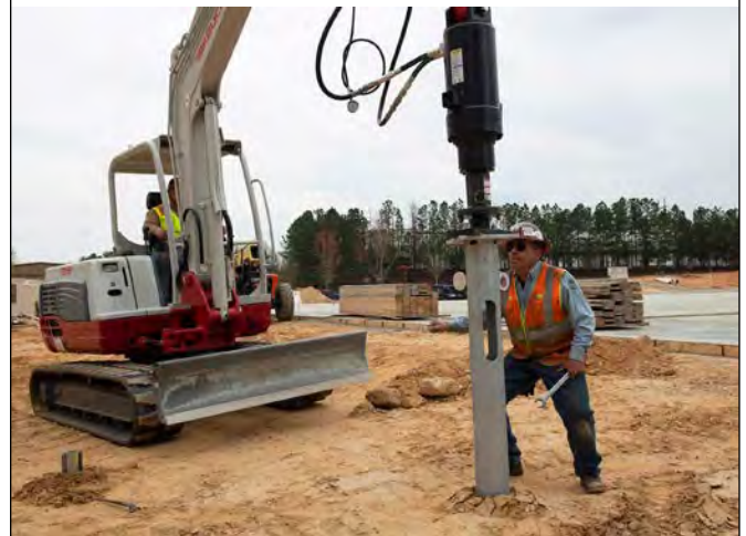
INSTANT FOUNDATIONS ARE INSTALLED USING COMMON CONSTRUCTION EQUIPMENT FIGURE 10-3
