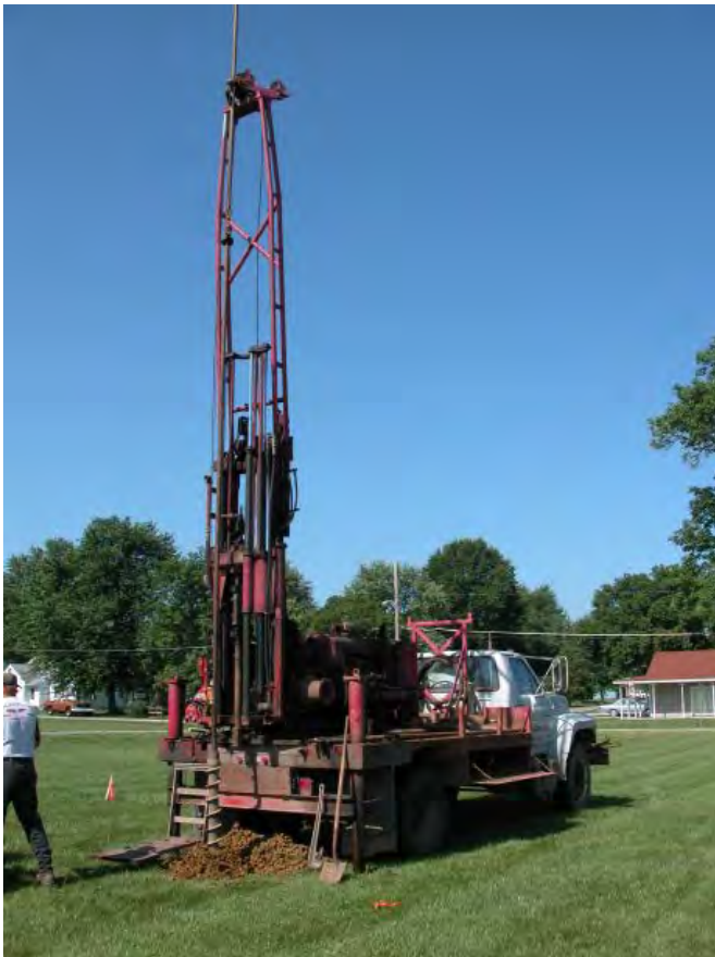
AUGER DRILLING OPERATION FIGURE 2-7
